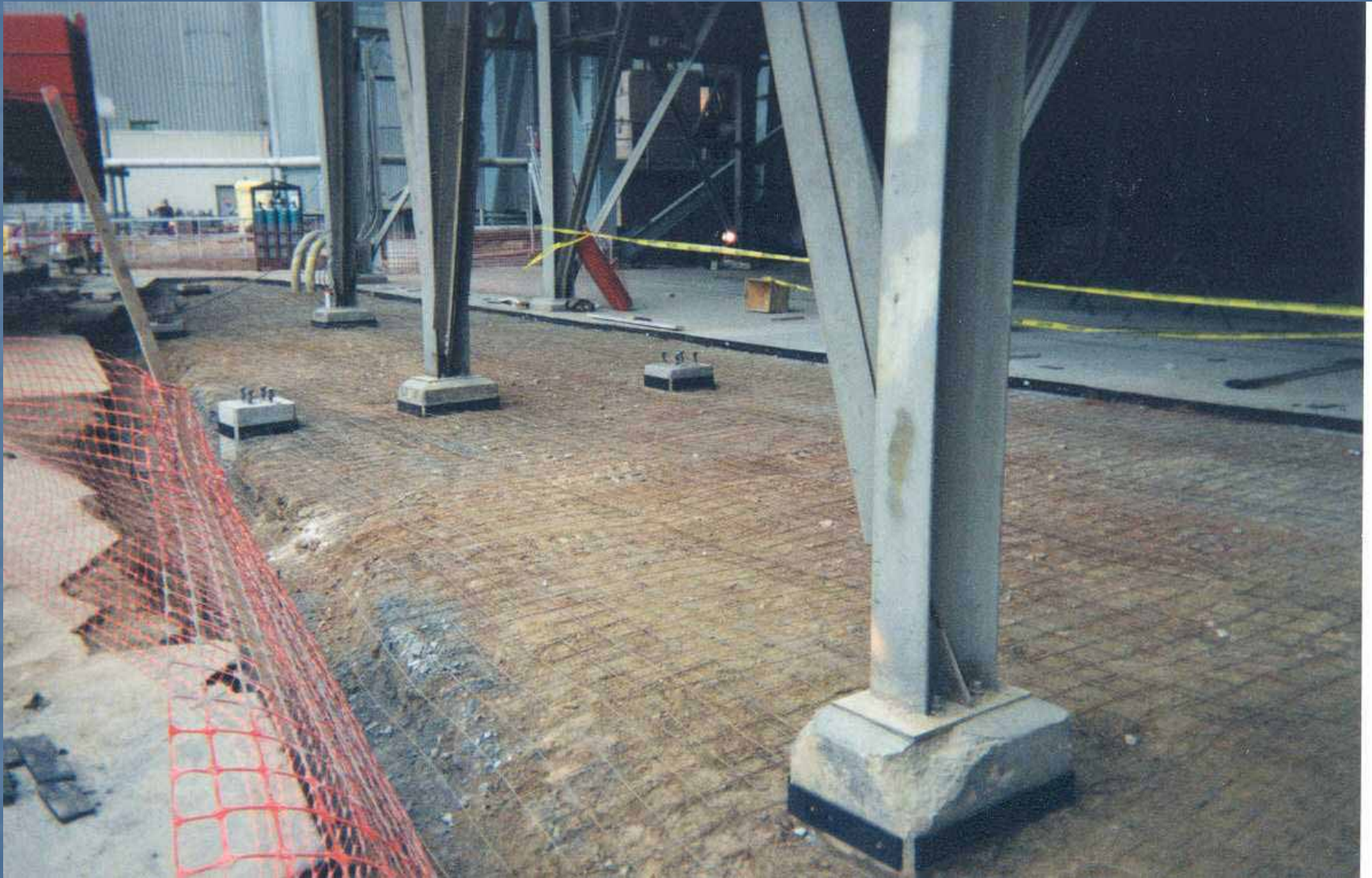
Prior to pouring Slab
